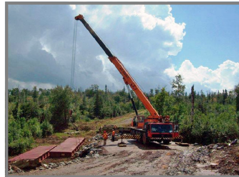
Installing a bridge!
